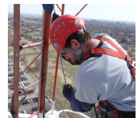
Wisper technicians installing a PTP radio on a tower.
