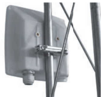
Installation on the mast
